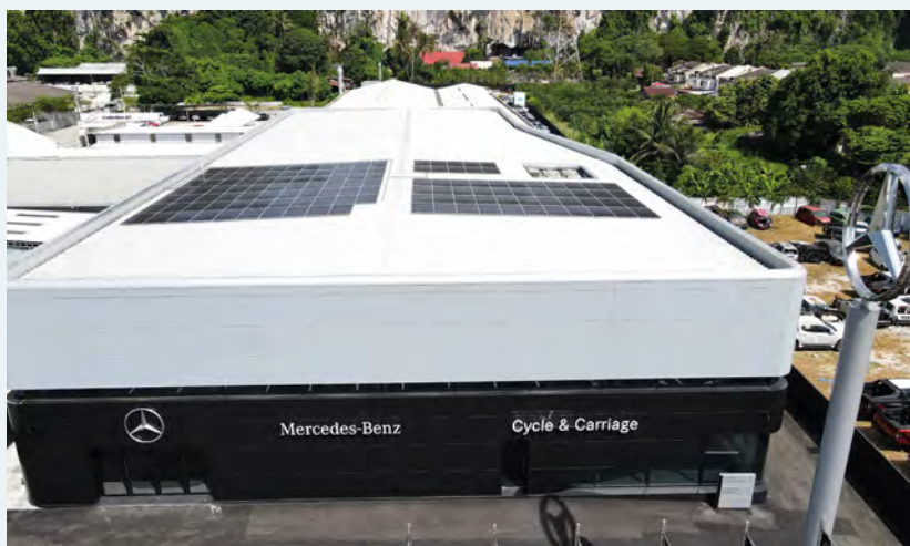
Rooftop solar at Cycle & Carriage Bintang Ipoh
