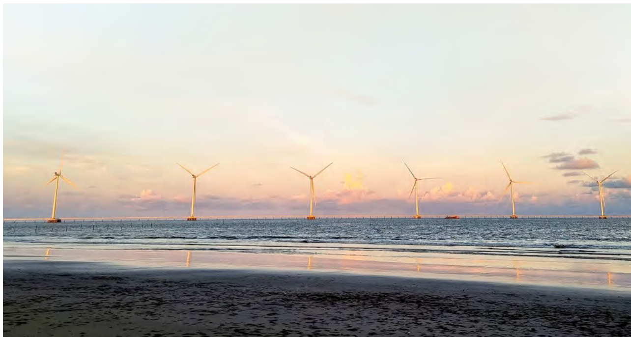
REE's Tra Vinh V1-3 Wind Power Plant
