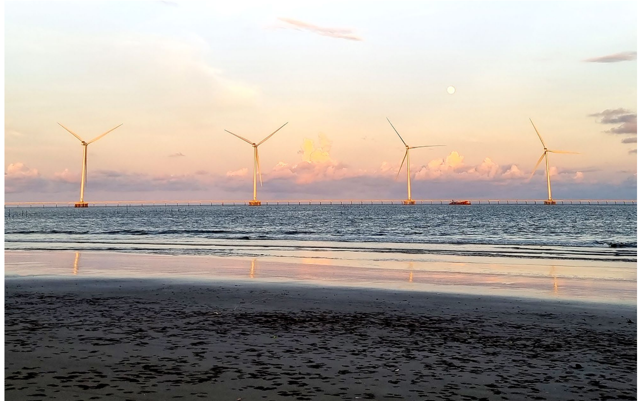
REE's Tra Vinh V1-3 Wind Power Plant
