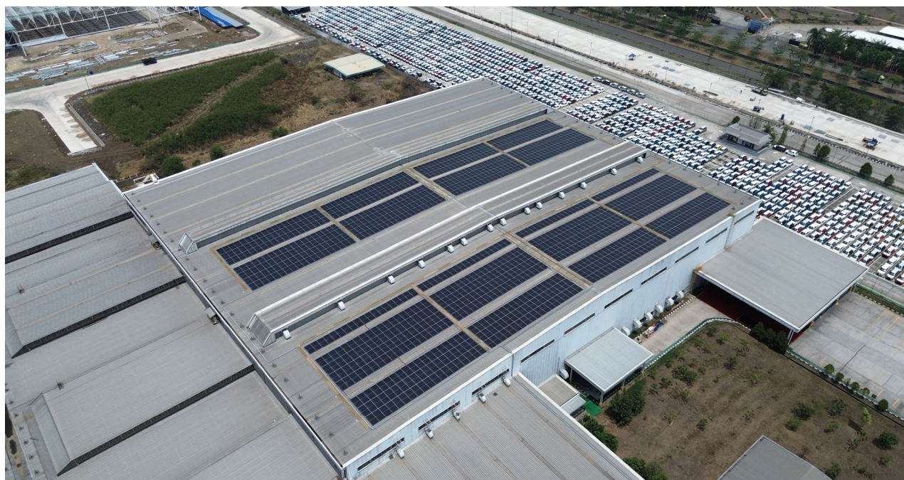
Solar panels at PT Astra Daihatsu Motor
