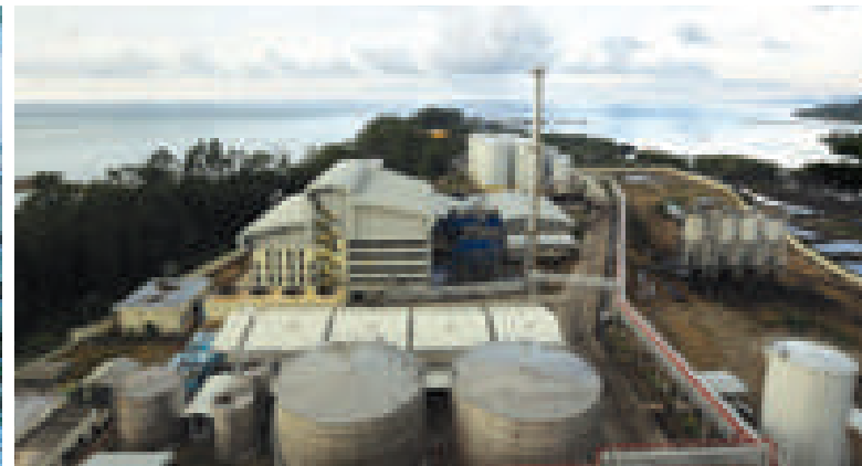
Palm Oil Refinery | Indonesia
